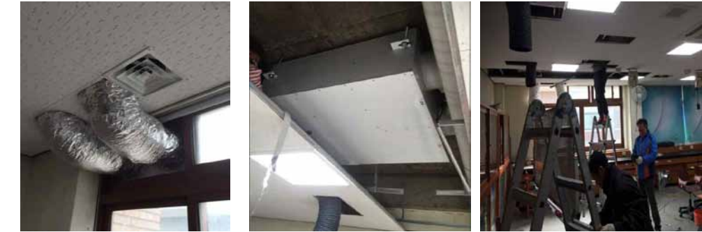
[Fig. 19] Construction of installing air ventilation system and waste heat recovery facility
