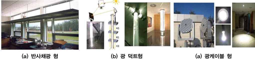
[Fig. 2] Types of solar lighting system
